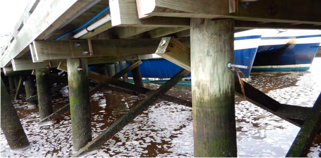
FIGURE 2-6: DPM MAINTENANCE FIXED PIER TIMBER PILE BENTS
